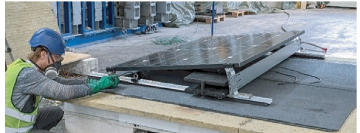
Figure 2 - Flat roof solar configurations. South facing configuration
